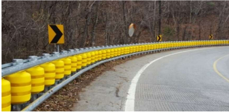
[Figure 5: Road Image with well-guarded barrier 3 ]
